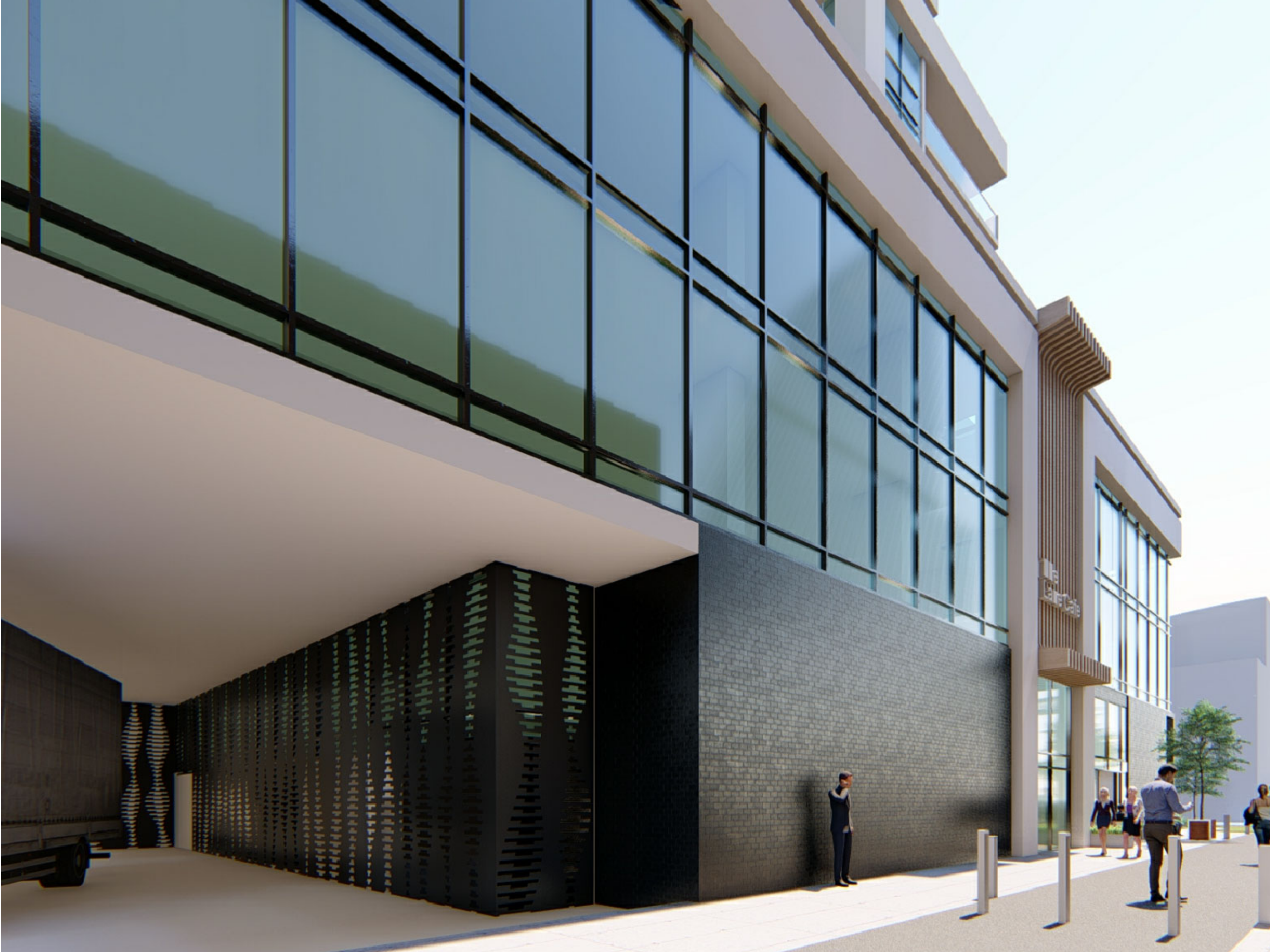
FUTURE LANEWAY & LOADING DOCK
